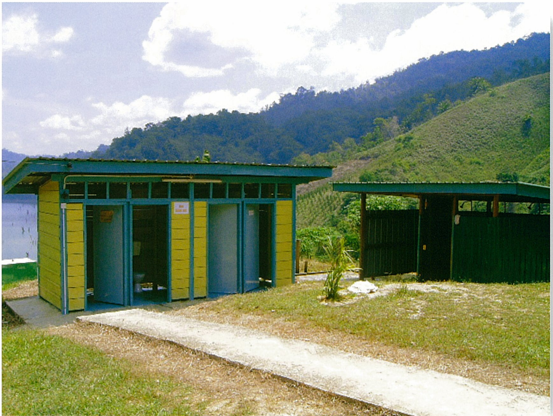
Toilets and shower room built for Nanga Delok Primary School.
